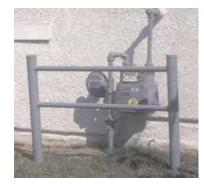
The Industrial Guard Post (left) is a medium duty barrier and the Residential Guard Rail (right) is a light duty barrier. Both are used to protect meter sets and/or regulator stations from vehicular traffic. The above ground portion of both is coated with a minimum of 2.5 mils polyester fusion coating.
